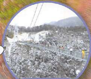
The bridge in winter
